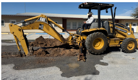
Pastor Tim Aguiar fixing the parking lot
